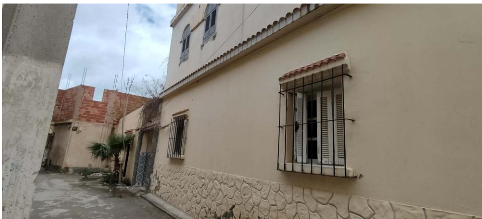
Figure S2: Ground-level view showing the adjacency of both models (Model No. 02 foreground, Model No. 01 background)
