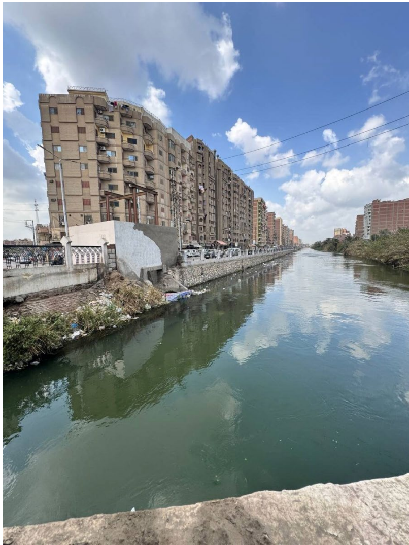
Figure I-4. El-Kased Canal at the raw water abstraction point, Tanta. The trapezoidal channel section shows the typical operational water level conditions. The intake structure for the post-upgrade system is visible on the left bank (Field survey, 2023).
