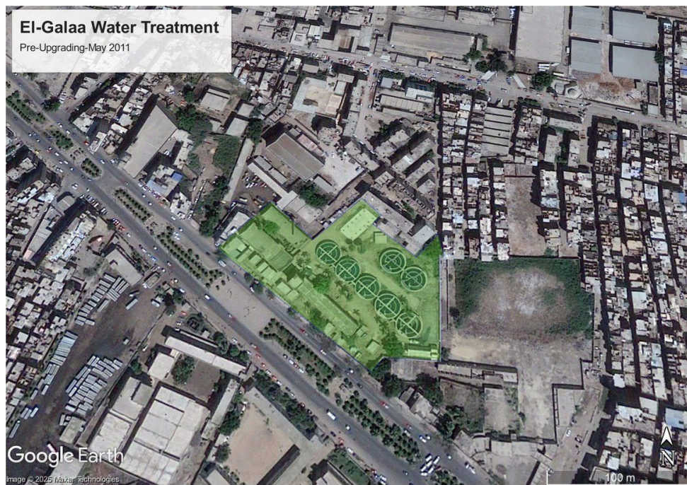
Figure H-3. Aerial satellite view of El-Galaa WTP, Tanta, prior to the 2019 modernization program. The image clearly shows the seven circular clari-flocculation units and six circular rapid sand filter vessels in their pre-upgrading configuration. The plant footprint and surrounding urban fabric are visible at 1:2,500 scale. Image source: Google Earth, image acquisition: May 2011, © Maxar Technologies.
