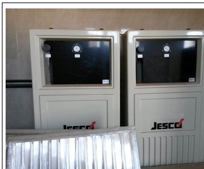
Fig. C-9. Two new JESCO gas chlorinator units (cream/grey fiberglass cabinets) prior to installation, still in delivery condition. Each unit houses a vacuum regulator, rate valve, flow indicator, and injector assembly within a weather-resistant enclosure. The dual-unit configuration provides full active-standby redundancy — a capability absent from the pre-upgrade system.
