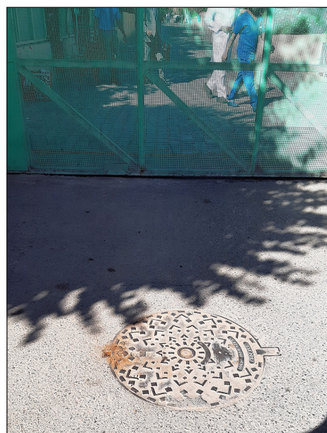
Figure 1. The main collector of effluents from the Mohammed VI University Hospital in Marrakech
