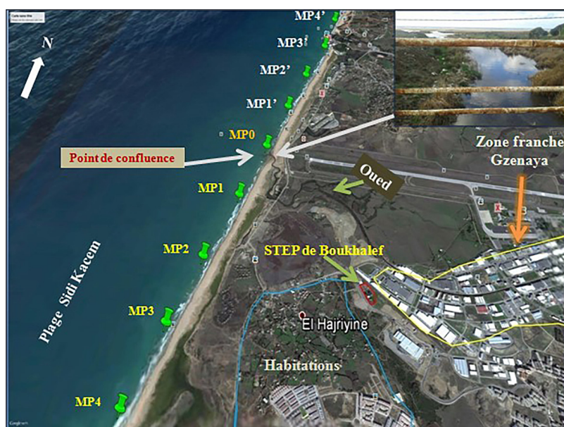
Figure 2. Sampling points for bathing waters at Sidi Kacem, the receiving environment for treated wastewater from the Boukhalef Treatment Plant in Tangier (www.maps.Google.fr)
