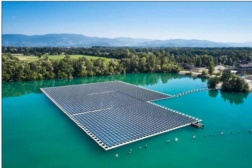
Figure 1. An FPV power plant with a net capacity of 749 kWp installed on Lake Maiwald near Renchen, Germany [23]
