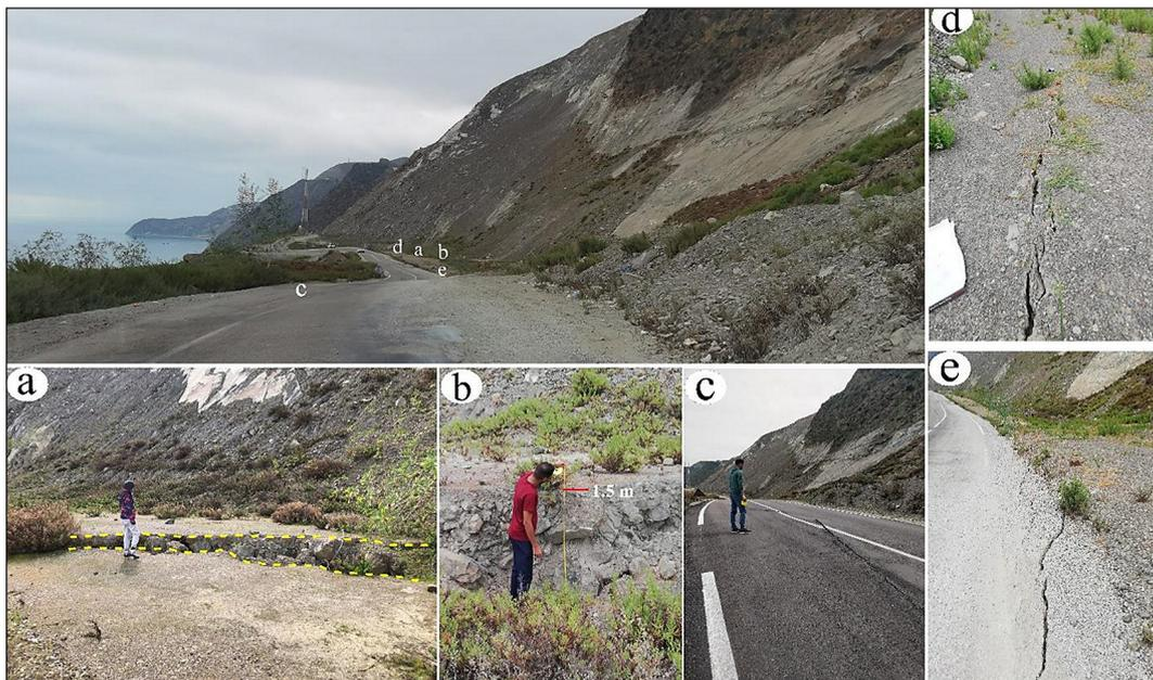
**Figure 9.** Illustration of some types of anomalies at the studied landslide during the field mission in 2023: (a) detached area, (b) subsided zone (~1.5 m), (c–e) the tension crack in the road and at bottom of the embankment
