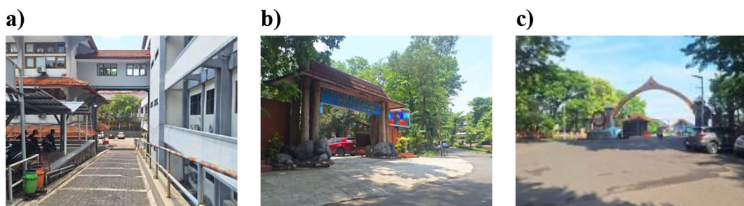
Figure 13. Some of the inundation-prone points in Zone C include: (a) FISIP building, (b) FEB gate, (c) access to the campus exit gate
