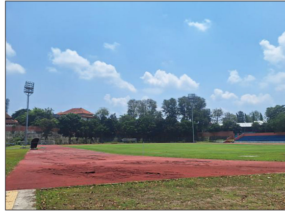
Figure 16. Inundation-prone points at UNS stadium
