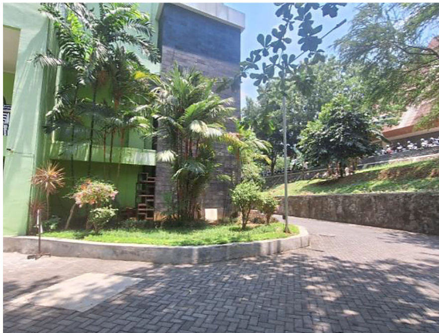
Figure 18. Inundation-prone points in the southern area of Javanologi
