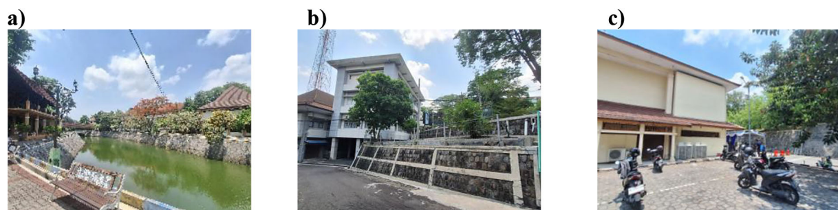
Figure 9. Some of the inundation-prone points in Zone A include: (a) UNS lake, (b) ICT building, (c) auditorium building
