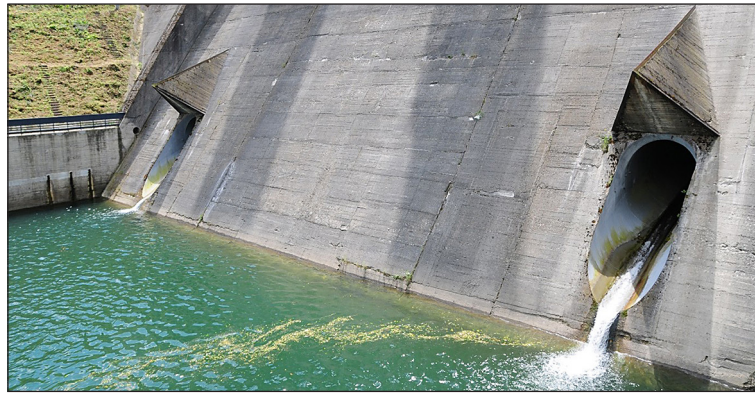
Figure 2. Bottom outlets of the Solina dam
