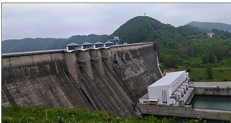
Figure 1. Spillways sections of the Solina dam
