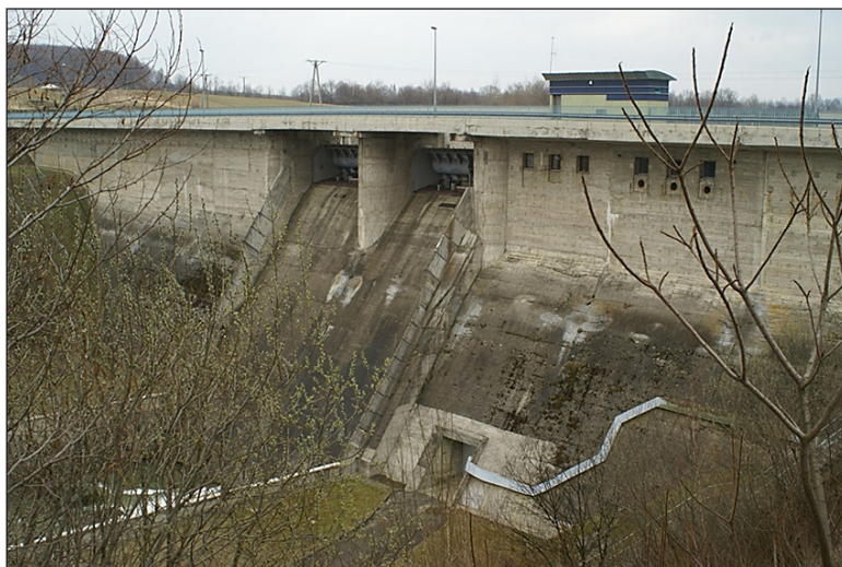
Figure 4. Spillway sections of the Besko dam
