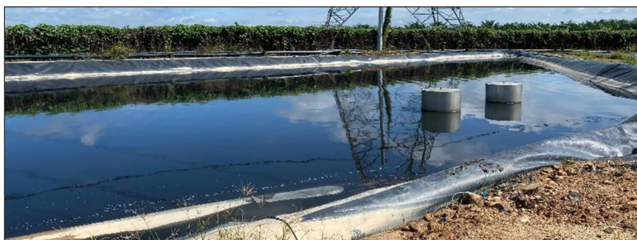
Figure 1. Actual photo of the leachate collection pond in Jeram Landfill, Selangor, Malaysia
