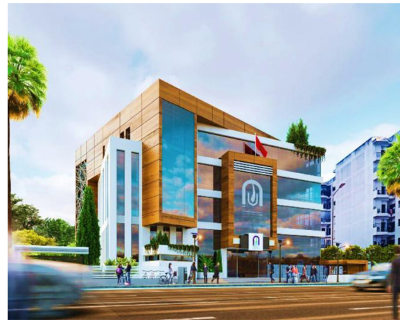
Figure 5. Architectural rendering of the AUKSS building exterior (Kenitra, Morocco), showing the north main façade, curtainwall glazing, upper-level wood cladding, and bioclimatic landscaping integration
