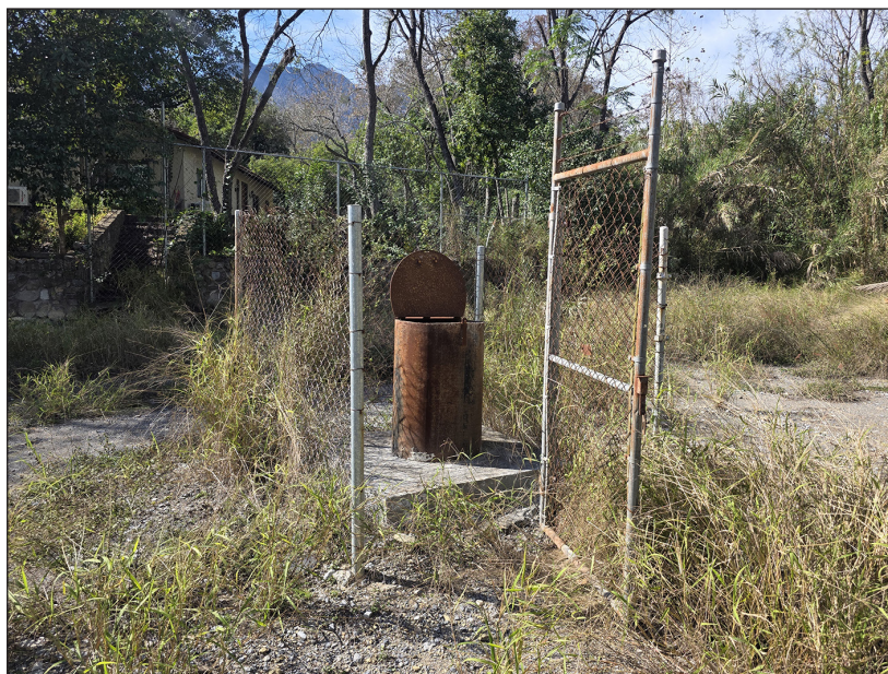
Figure 13. Surface structure of the recharge well used for stormwater injection at the Galería Los Elizondo site
