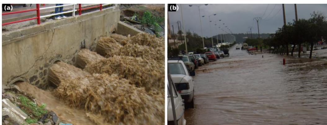
Figure 2. Flooding of 26 January 2010 at the RN16 crossing: (a) high-velocity outflow at the five-culvert structure; (b) submersion of the RN16 roadway
